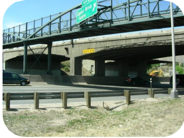
Image 8: South Elevation View of Speer Blvd Southbound over I-25 (E-16-E0)
