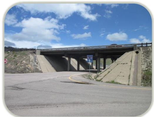
Image 2. Existing I-25 SB over County Rd (H-17-CI)
