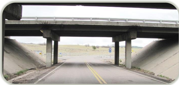
Image 1. Existing I-25 NB over County Rd (H-17-CH)
